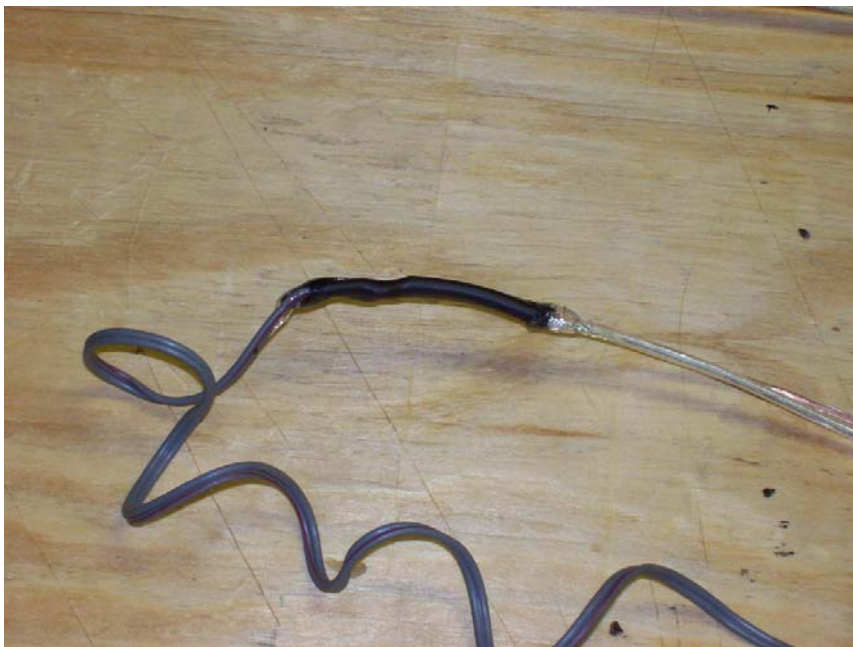
Seal and waterproof the wiring splice with glue.
